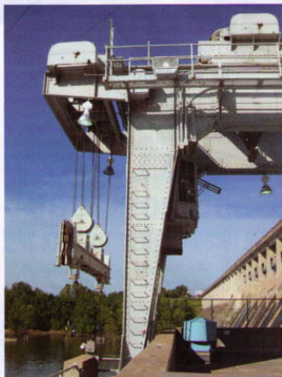
Right: The power house crane in the foreground, and the houses for the two gate cranes above
